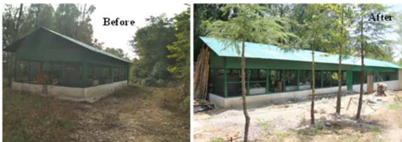
Bamboo treatment plant
