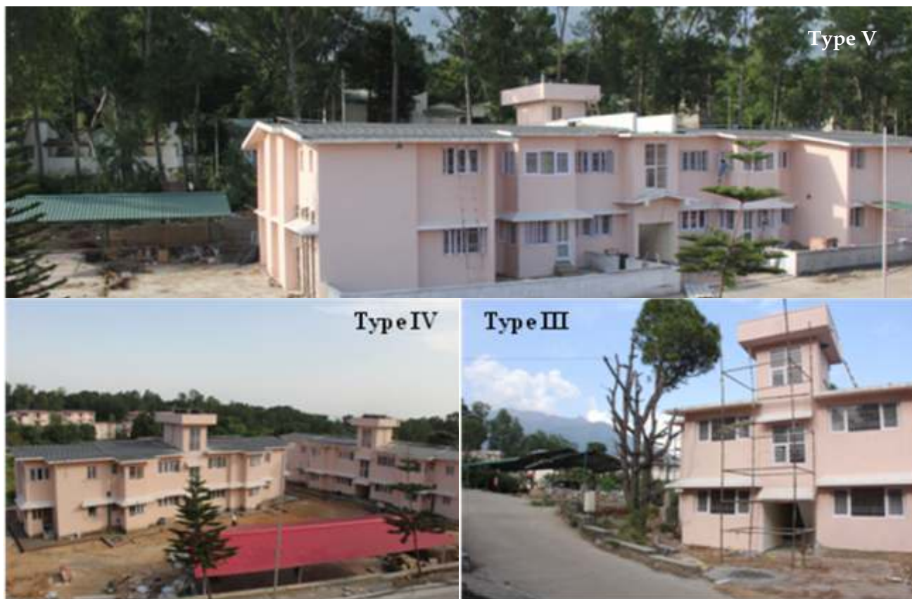
Construction of staff quarters
